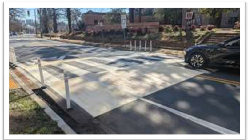
Figure 34 Crosswalk visibility enhancements 26
